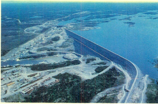
CMC's mobile radiotelephones and base stations provide an important network of vehicle, aircraft and fixed communications for the James Bay hydro-electric project.
