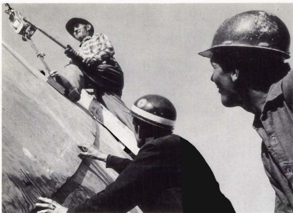
Speeding the completion of Manic 2 — At work on a draft tube form.
