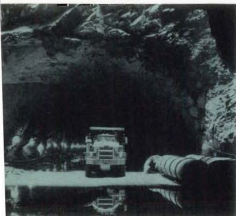
Diversion tunnels are cut through the mountain.
