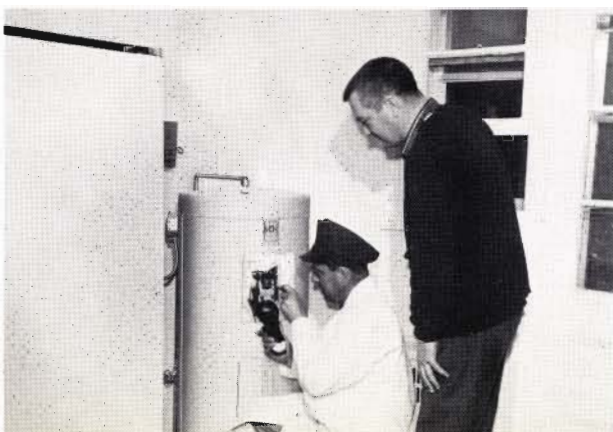
Testing the installation of an electric water heater under Hydro-Quebec's rental plan.
