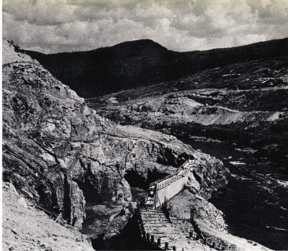
Bird's eye view of the Manicouagan 5 construction site.
