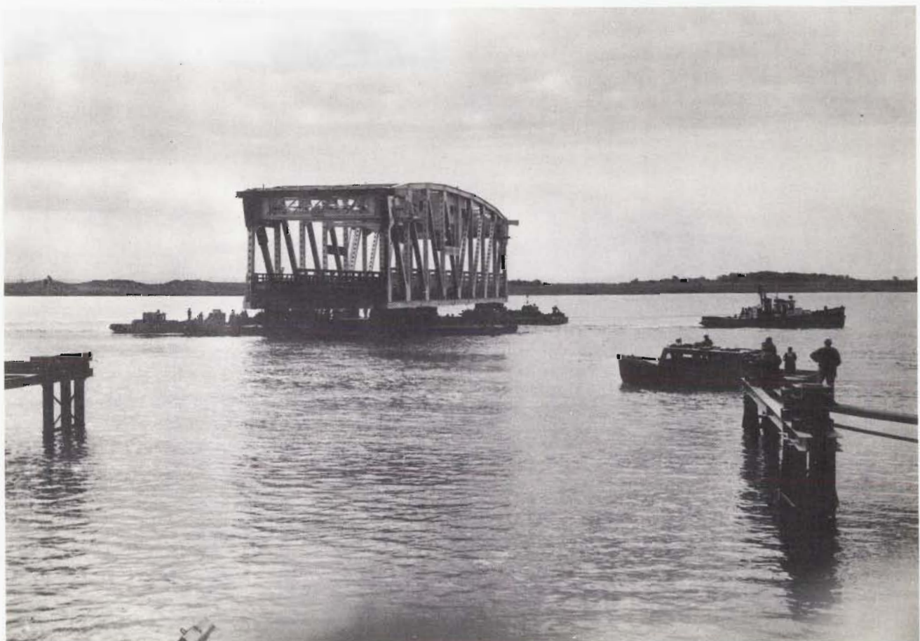
Delicate operation by construction crew at Beauharnois
