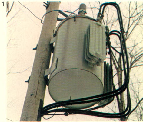
1 Transformer mounted on a hollow concrete pole.
