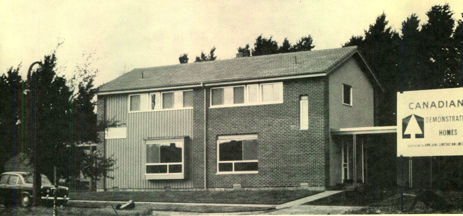
Demonstration houses at Abbots Langley, near London, England, designed and built by the Corporation for the Department of Trade and Commerce, Canada. Three exterior finishes are employed — board and batten, brick and stucco — to illustrate the flexibility of Canadian construction techniques.
