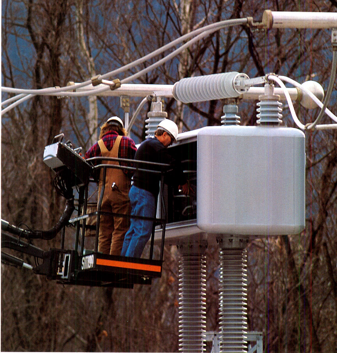
This outdoor thyristor switching device, the first of its kind in the world, is part of a new technology which allows a higher level of power to be maintained on existing lines. The equipment is located at an Appalachian Power Company switching station near Charleston, West Virginia, USA.
