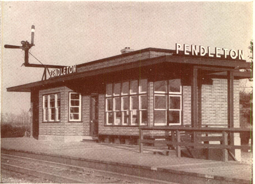
The station at Pendleton, Ontario, is the first in a series of new style depots incorporating modern design and improved facilities.
