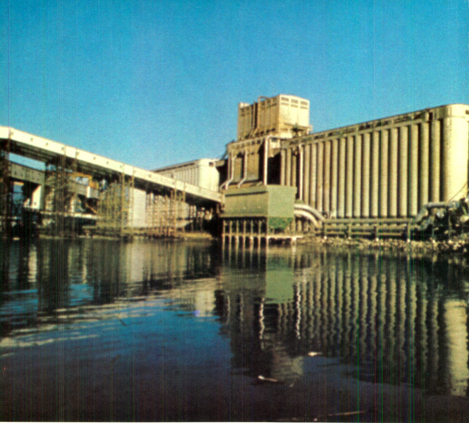
New centralized bag house (square building on stilts) is the heart of new dust control systems at Alberta Pool's Vancouver terminal.
