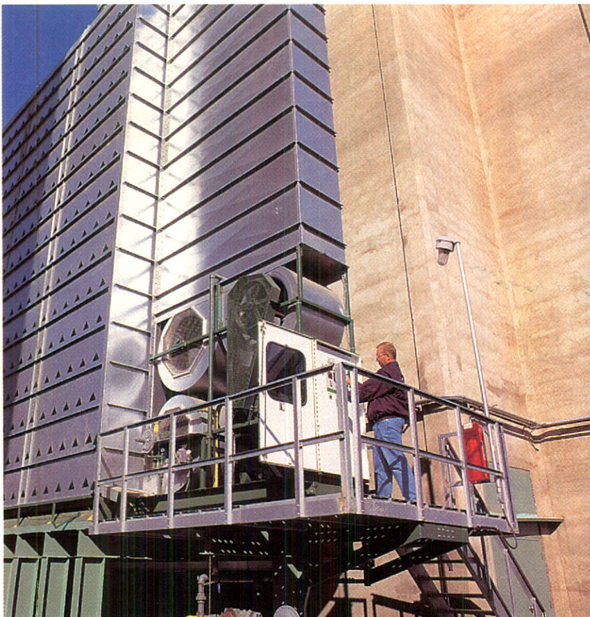
High speed grain dryers at Alberta Pool's Legacy Junction and Smoky River facilities can handle 3,000 bushels per hour, providing the opportunity for early harvesting and better grades.
