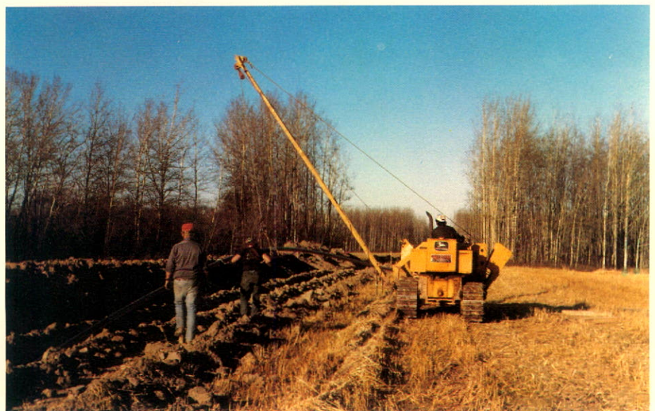
Laying gathering line
