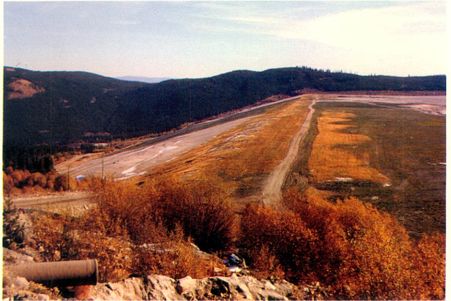
New vegetation growing on the tailings dam, resulting from the seeding program.
