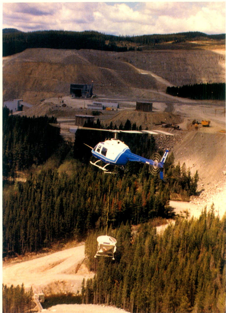
The reclamation program includes the use of a helicopter to seed the tailings dam.
