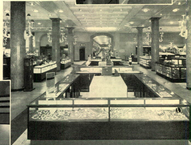
GENERAL VIEW Main Floor
