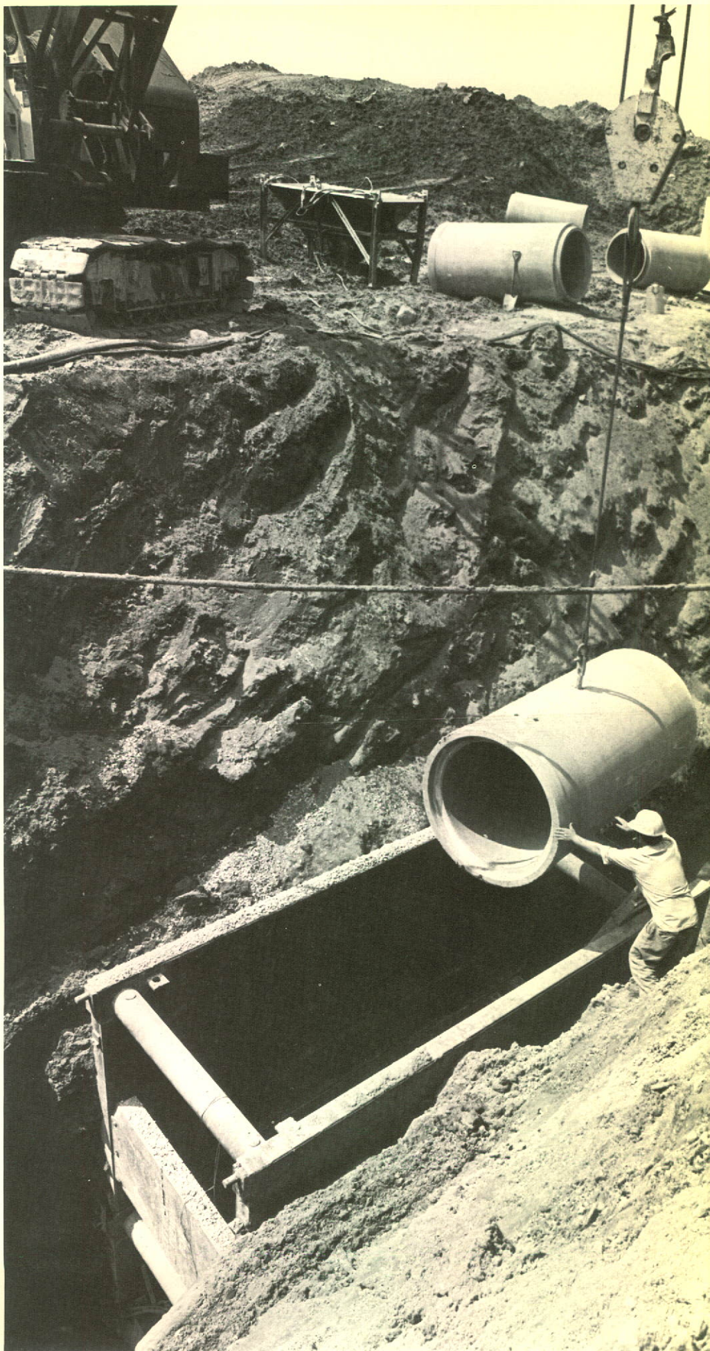
Trunk sewer installation in Amberlea, Town of Pickering, Ontario
