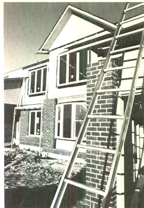
Residential Construction, Pickering, Ontario
