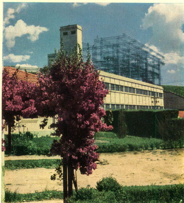
PEDREIRA PUMPING STATION WHICH PUMPS WATER TO THE BILLINGS RESERVOIR TO FEED THE SERRA DO CUBATÃO PLANT.
