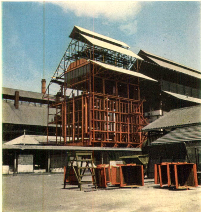
NEW RETORT STRUCTURE FOR THE GAS PLANT IN RIO DE JANEIRO.
