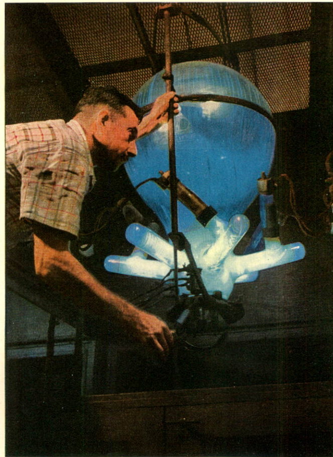
ONE OF THE MERCURY ARC RECTIFIERS PROVIDING DIRECT CURRENT FOR STREET RAILWAYS.
