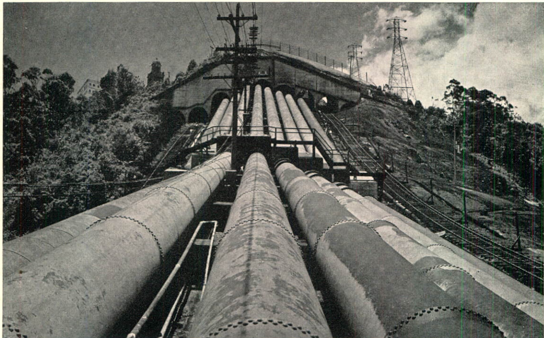
CUBATÃO GENERATING PLANT—VIEW OF PENSTOCKS.
