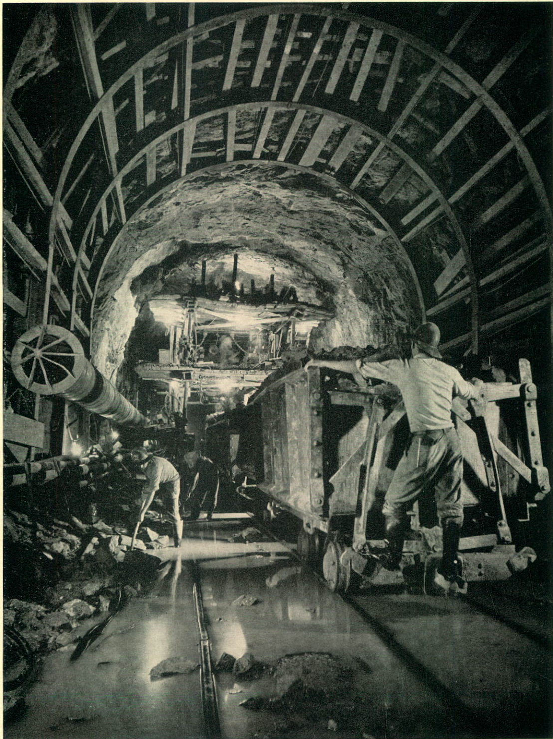
SANTA CECILIA TUNNEL—NORTH HEADING 6 DAYS BEFORE HOLING THROUGH.
