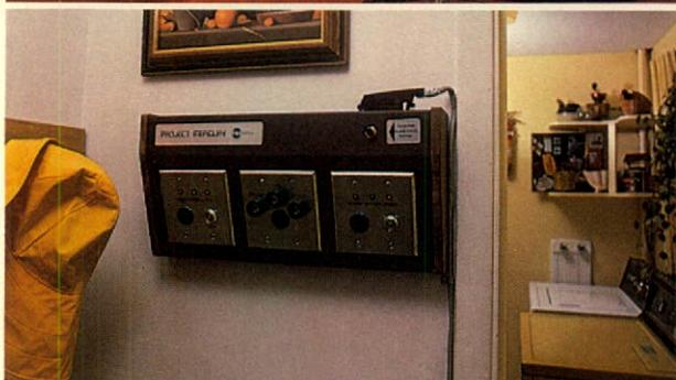
Residential security is just one part of the company's Project Mercury field trial now taking place in Saint John. This control panel contains switches which allow users to instantly summon police, fire and medical authorities. The panel also controls an elaborate intrusion alarm system.
