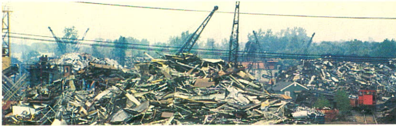
June 11, 1983 — a critical 10 day demolition phase began. An army of demolition experts armed with acetylene cutters removed 18,350 cubic metres of scrap which filled 325 railway gondola cars and 420 tandem-axle dump trucks.
