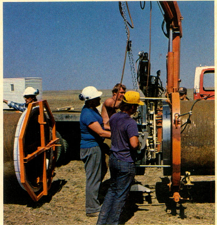
Pipeline welding using explosives is a new development described on page 19.
