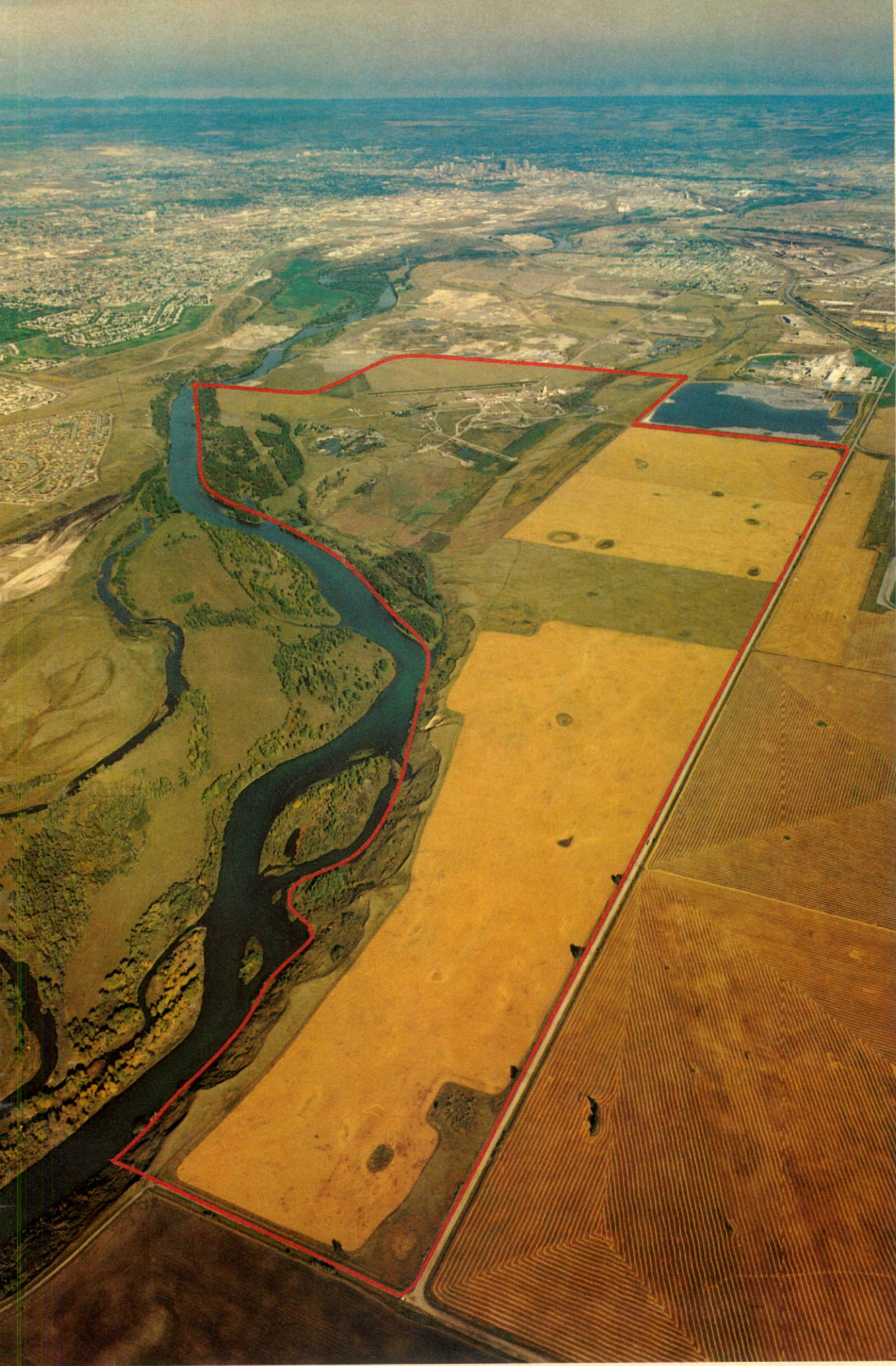
In southeast Calgary, about 1200 acres of property will be developed for residential, commercial and industrial use by C-I-L subsidiary, Douglasdale Estates Ltd.
