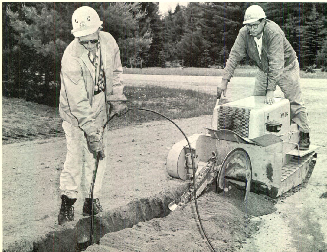
More and more telephone cable of all kinds is being placed underground. This trencher is burying the cable to bring service to a new home in the Madawaska Valley, north of Belleville, Ontario.
