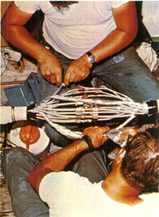
Splicing LD-4 cable at Northern Electric's wire and cable division. The system can accommodate 20,000 two-way voice channels on a 12-tube coaxial cable.
