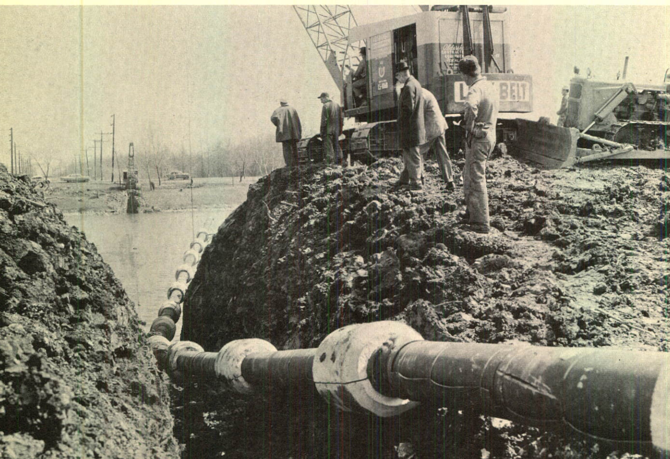
This air-tight, steel pipe, buried in a trench under the bottom of the Welland Canal was installed in 1963 to protect submarine telephone cables from ships dragging their anchors.
