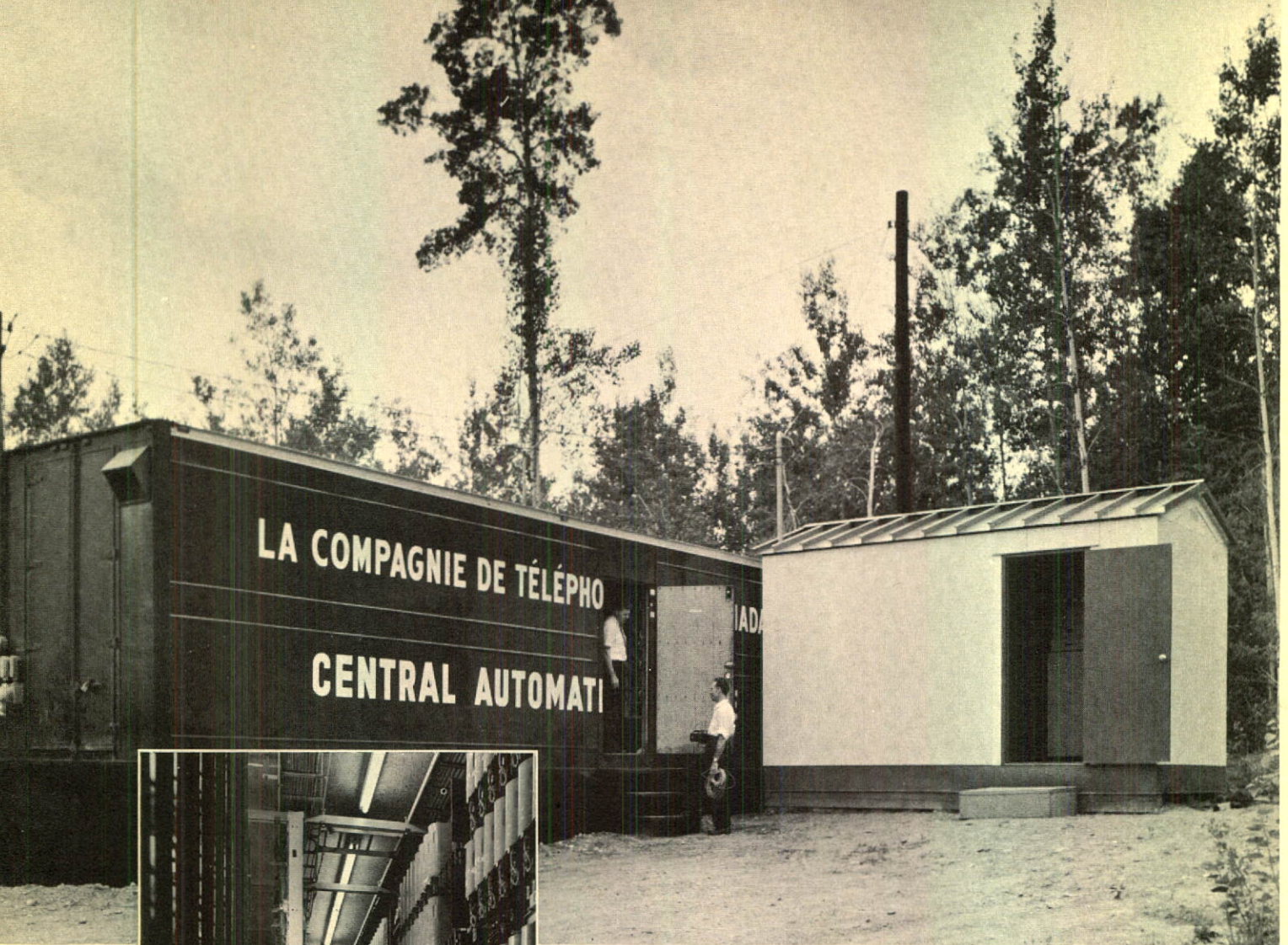
Dial service came on wheels to Shebandawan, in northwestern Ontario, during 1963. This mobile central office serves the community pending installation of a permanent one. Inside the van, a technician tests equipment.
