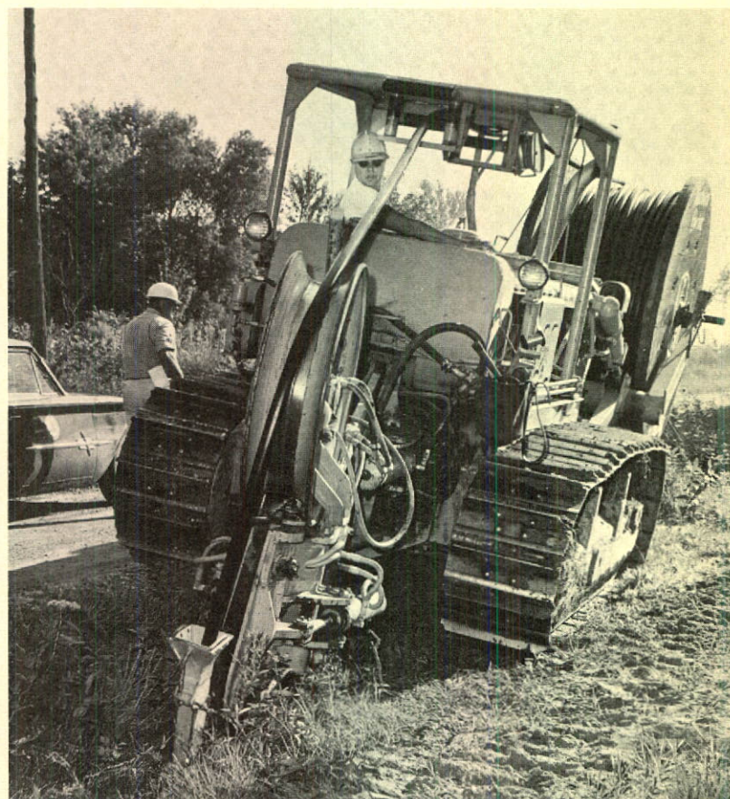
This heavy equipment buries cable near Tillsonburg in preparation for extension of the Tillsonburg-Otterville calling area.
