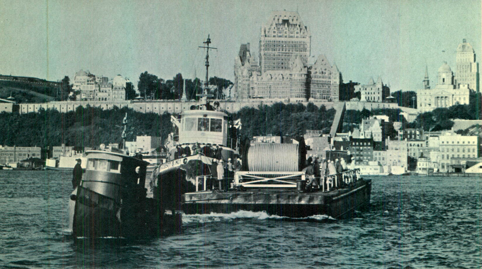
Construction crews place another large cable on the St. Lawrence River bottom between Quebec City and Levis. Press, radio and television representatives are on hand to report the event.
