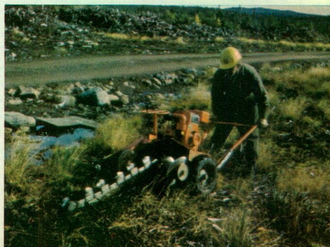
This employee uses a light, air-transported power tool to make a trench for the laying of buried cable at Cartwright, Labrador.
