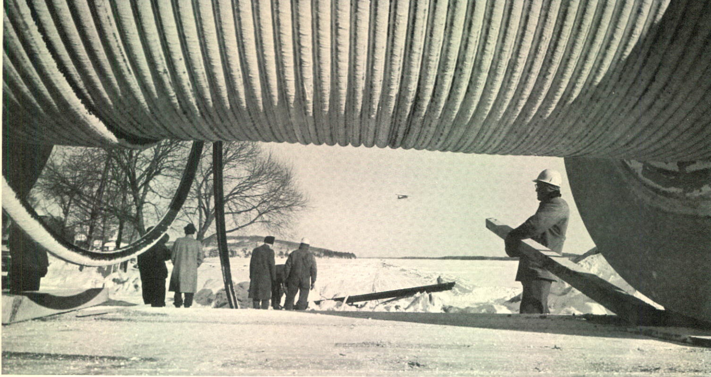
Working in temperatures of 40 below zero, construction crews cut through two feet of ice to lay this submarine cable across a lake in northern Ontario.
