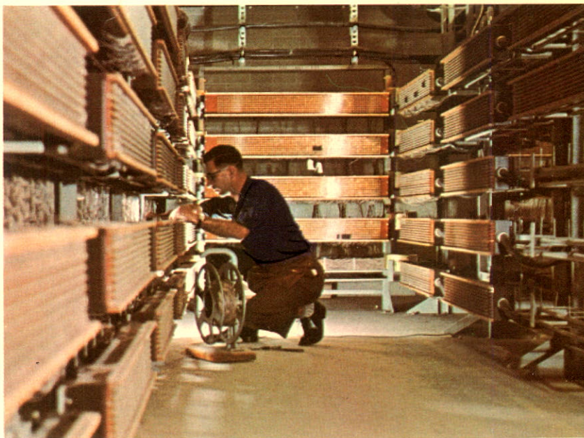
COMMUNICATIONS NERVE CENTRE of Place Ville Marie is this specially constructed, air conditioned room from which wires in their thousands fan out to telephones throughout the complex. Massive cables link the centre with a nearby Bell equipment office.
