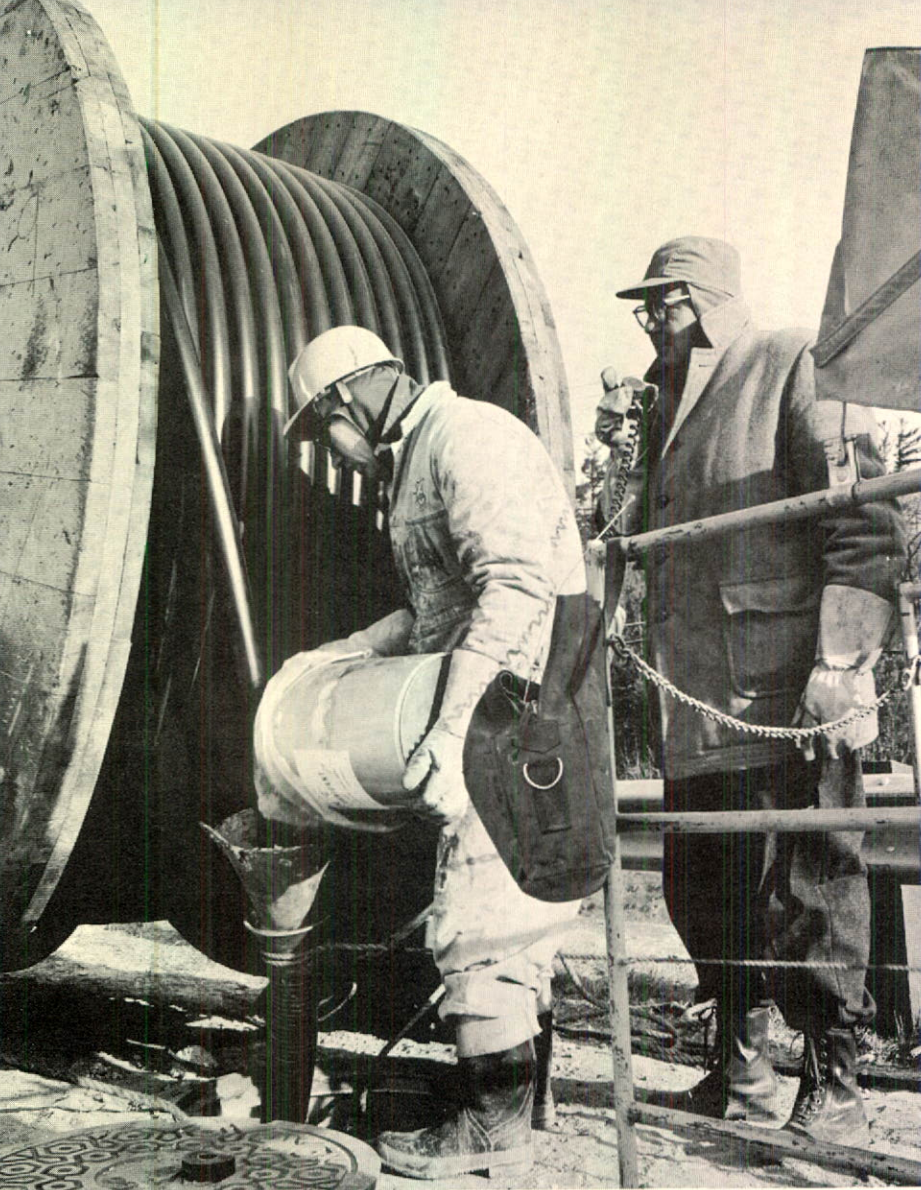
Extra-long cables, carried on massive reels like the one pictured here at Islington, Ontario, speed the job of placing cable underground. Crews keep in touch by portable radio.
