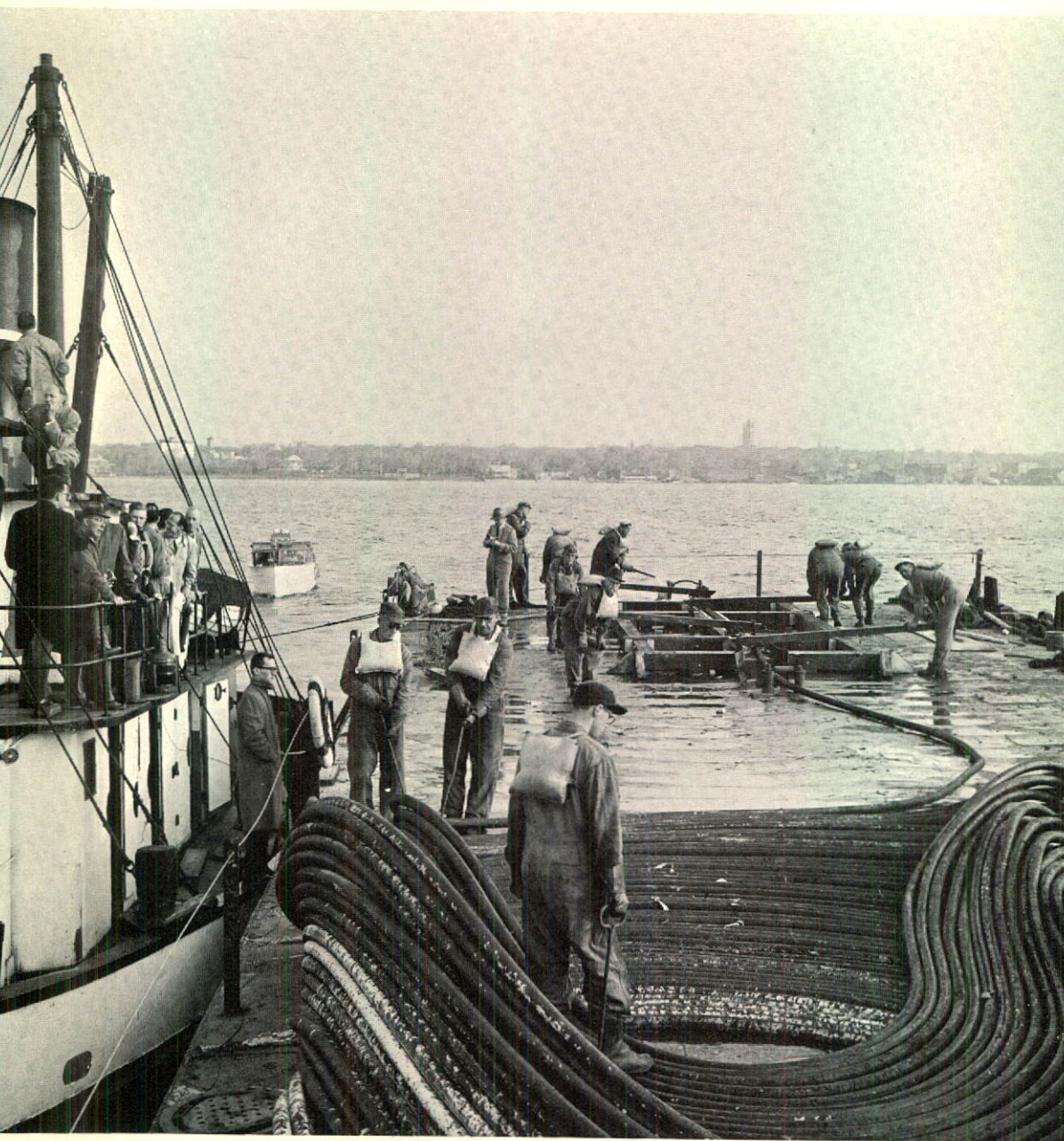
This 14,300 foot submarine cable was laid in the St. Lawrence River between Kingston and Wolfe Island. The fast-moving operation, using two tugs and a cable-laying barge, took just three hours to complete.
