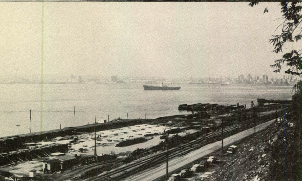
Good progress is being made on construction of Saskatchewan's Pool new 5,300,000-bushel terminal at Vancouver. Top photo shows workhouse rising above tideflats on North Shore. Excavation in foreground is basement of trackshed; middle picture shows concrete footings to carry grain tanks of east annex, piling and reinforced concrete below footings support the structure; bottom shows reinforced concrete slab poured on footings to support west annex. Photos were taken October 14, 1966.
