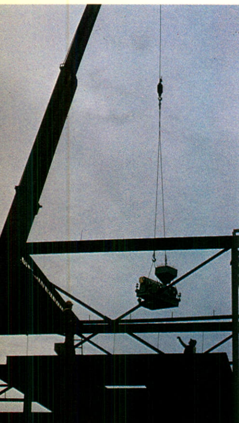
The warehouse roof at CB Packaging was raised in order to install the co-extrusion system.
