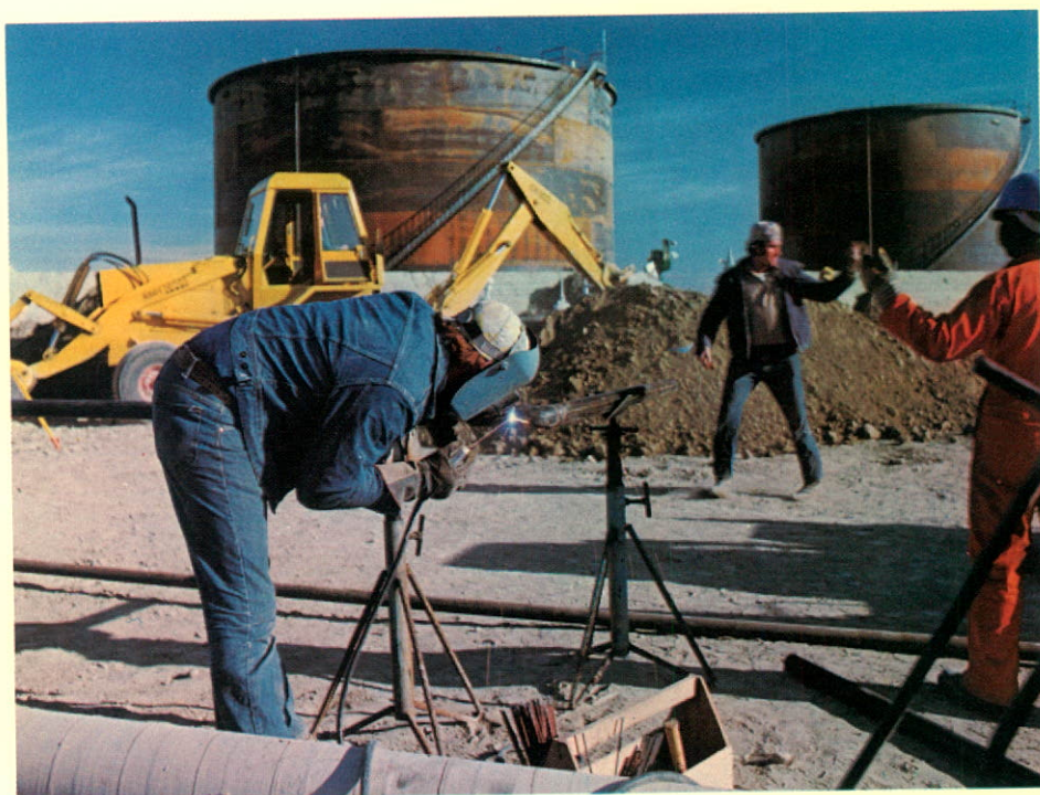
Construction of Alberta Products Pipeline facilities at Calgary International Airport. The new line permits the movement of jet fuels directly from Edmonton refineries to the airport.
