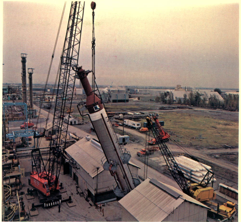
Hundred-foot tower is lifted into place as part of catalytic reformer expansion at Montreal plant.
