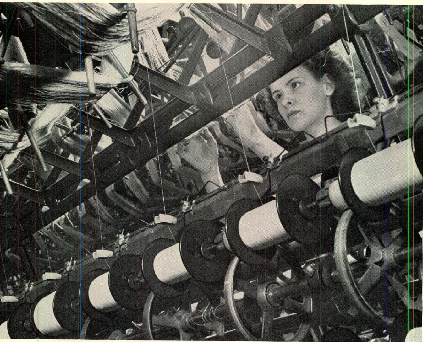
Watchful eyes follow the threads from hank to spool. This is one of the primary operations in the manufacture of Bruck Fabrics.
