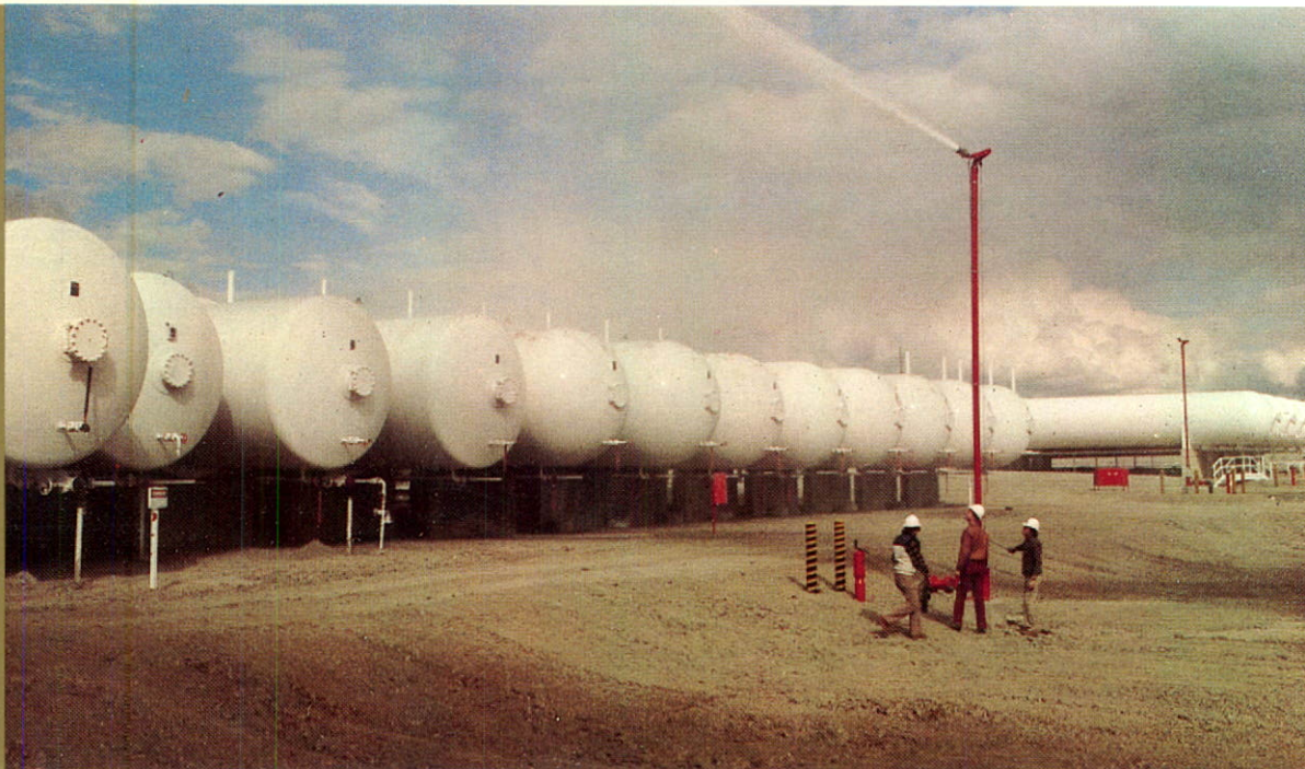
Water flow tests are conducted at natural gas plant (left) in the U.S. state of Wyoming.
