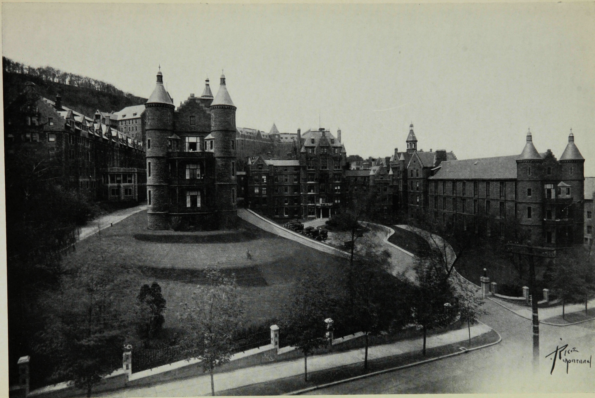
THE ROYAL VICTORIA HOSPITAL (MAIN BUILDING)
