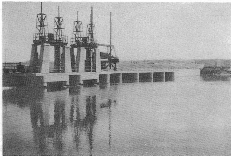
LOOKING DOWN RIVER—NEW DAM— LOWER METIS
