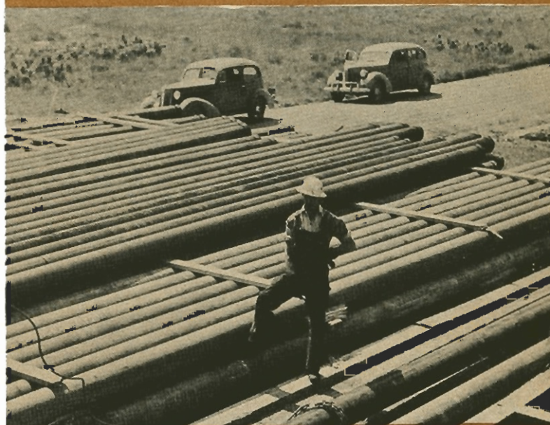
More than a mile of casing is needed to line a Turner Valley well
