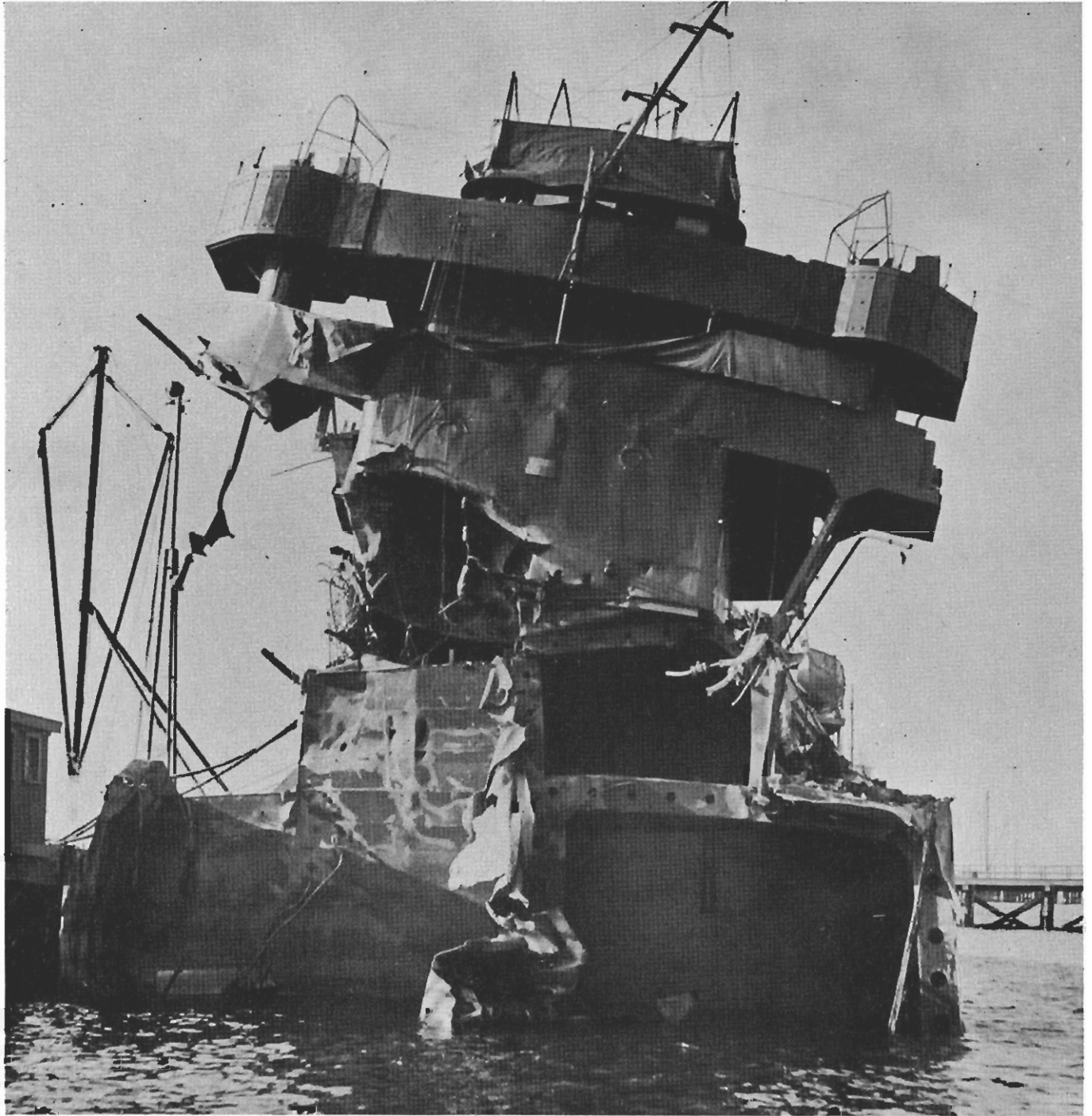
In port and afloat! What happened a tanker in an encounter with the enemy is shown here. Although the ship was blown in two the after part was saved to sail the seas again with a new fore part.
