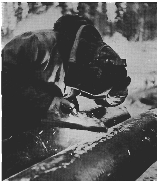
Many trades and crafts are employed by Imperial Oil. Above a welder joining two sections of pipe line. Modern welding practices greatly speed pipe line construction.
