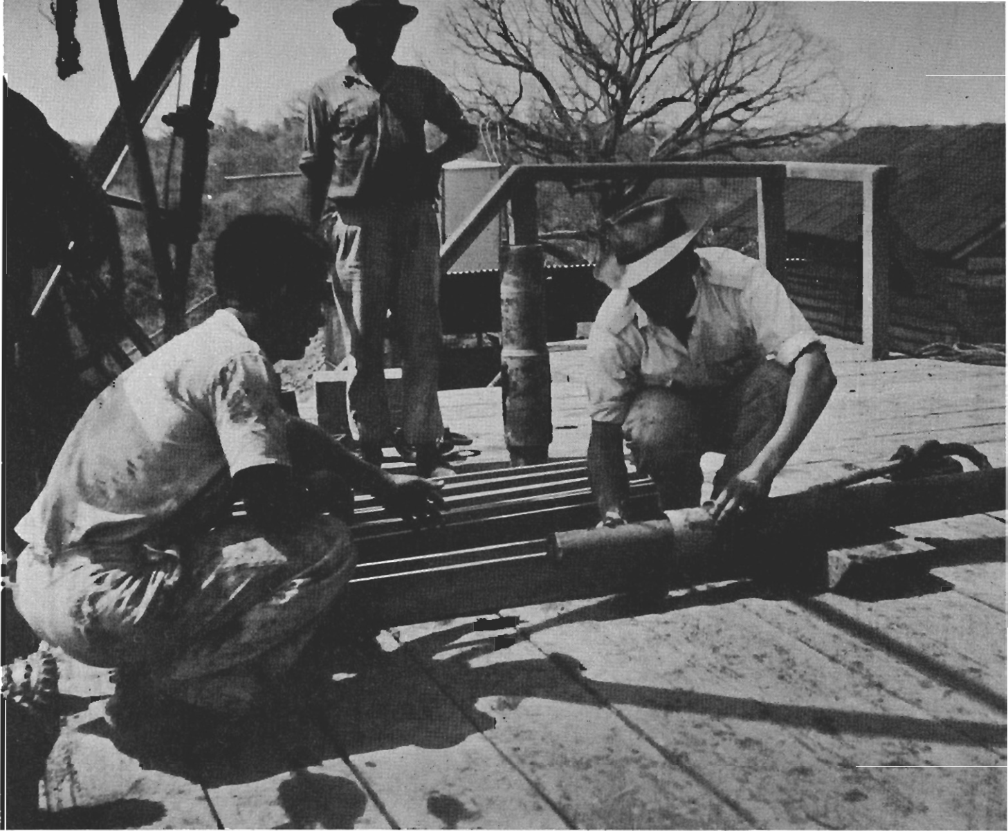
Extracting core from core barrel at an exploratory well in Ecuador. This core was cut at a depth of 6,030 ft. and provided the geologists with a sample of the formation penetrated at that depth.
