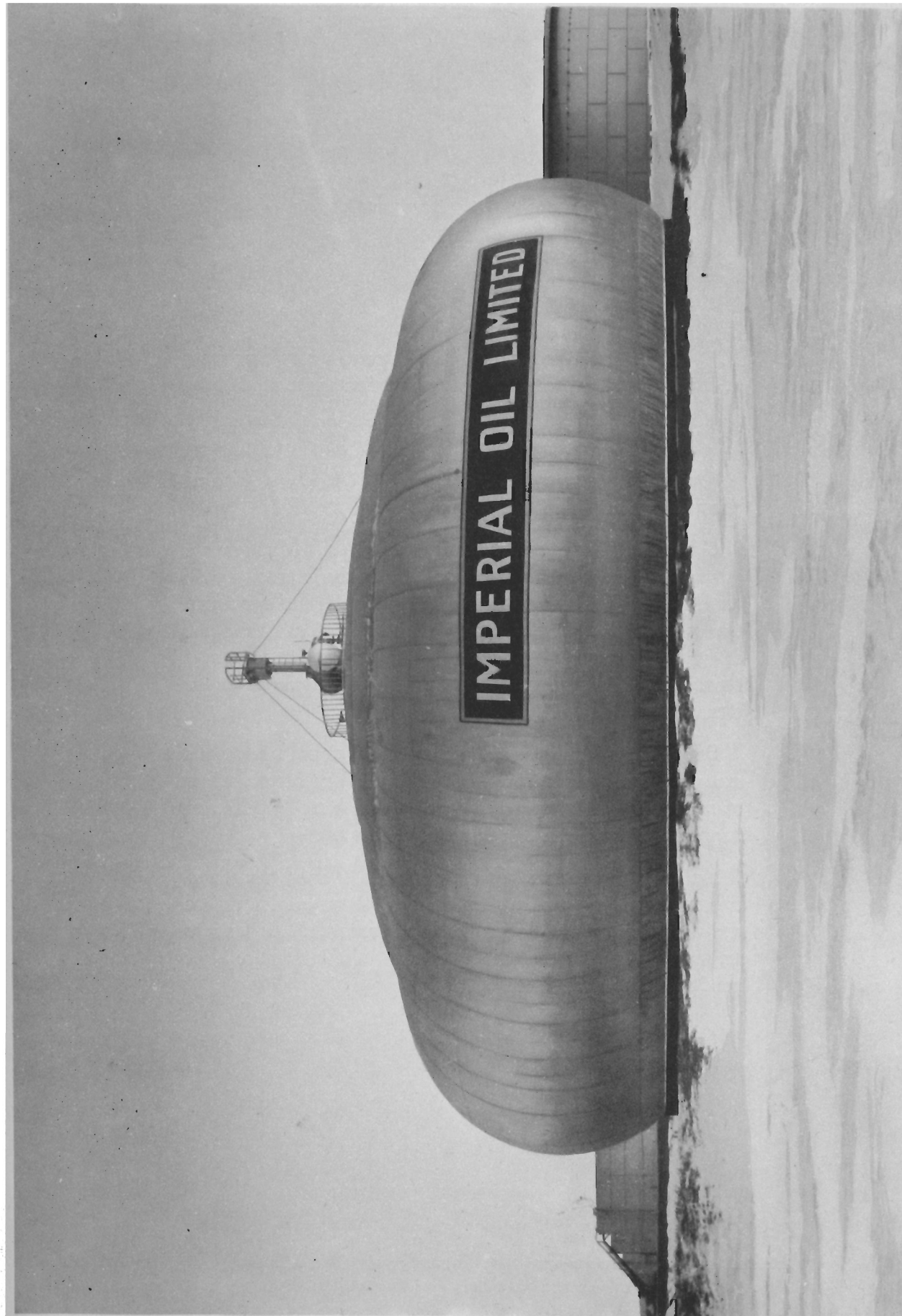
MONTREAL REFINERY • Spheroid pressure type tankage of 100,000 barrels capacity typical of new construction for storage of volatile products where the minimizing of losses is important from the standpoint of both conservation of quantity and quality.
