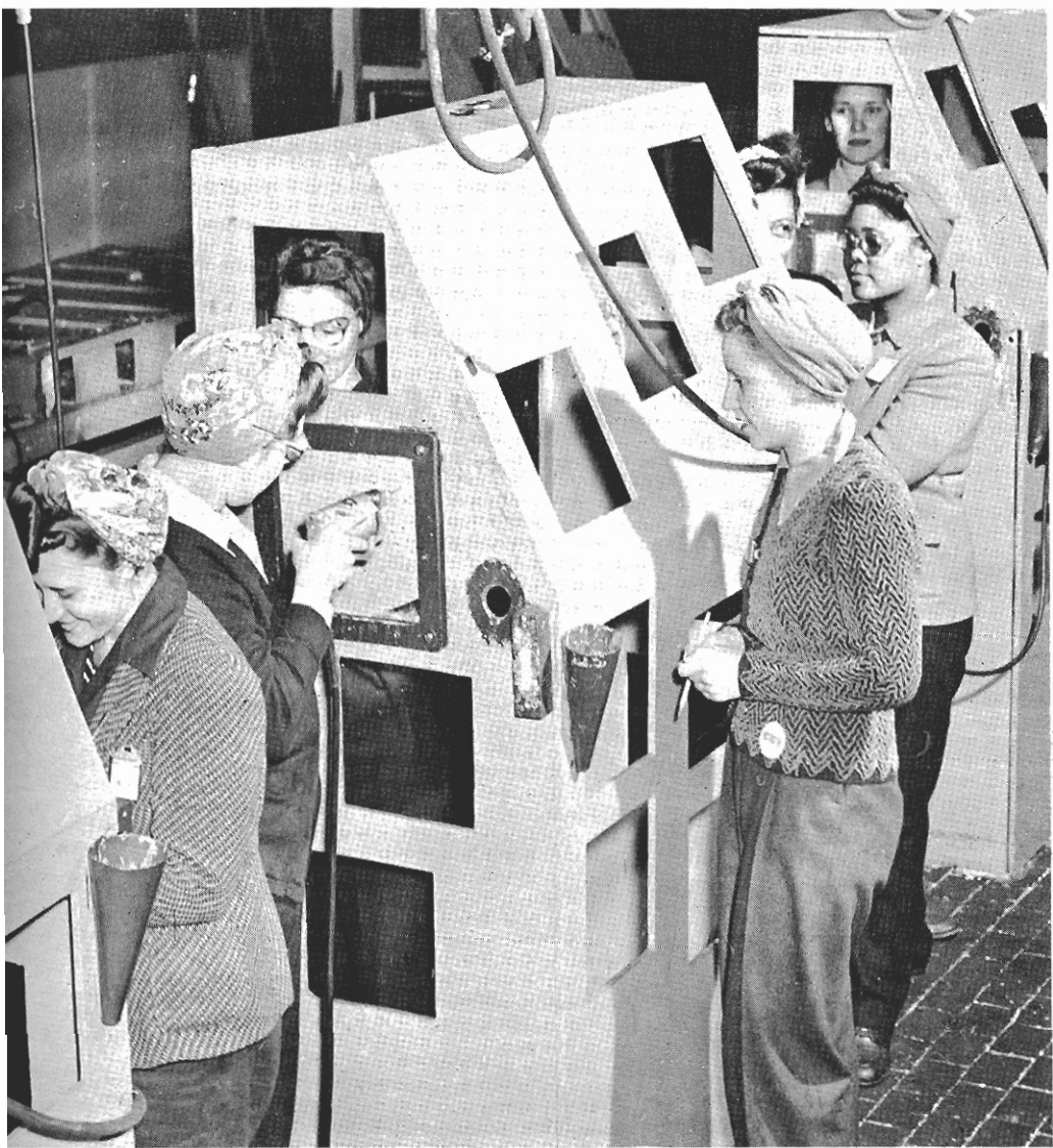
Many thousands of women are employed in war production in the various divisions of General Motors. Here trainees are learning techniques in airplane construction at Eastern Aircraft Division.
