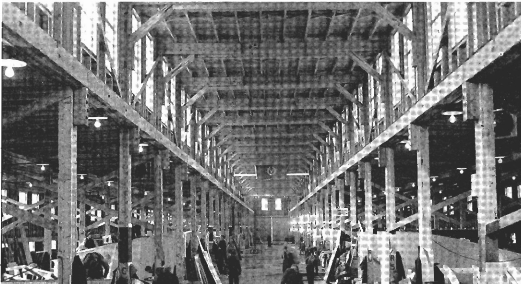
AN ERECTION AISLE.—BRIDGEWATER PLANT, FOUNDATION MARITIME
