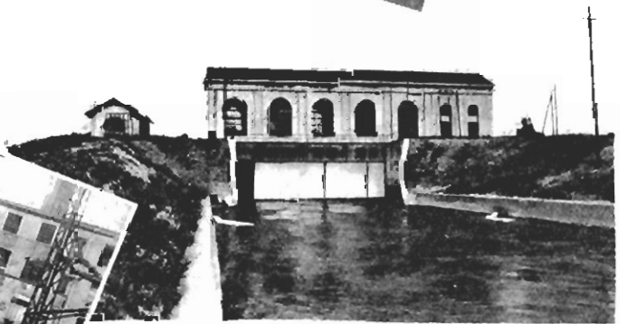
ABOVE Power House at Chatelot, Société Electrique de Bel- champ.
