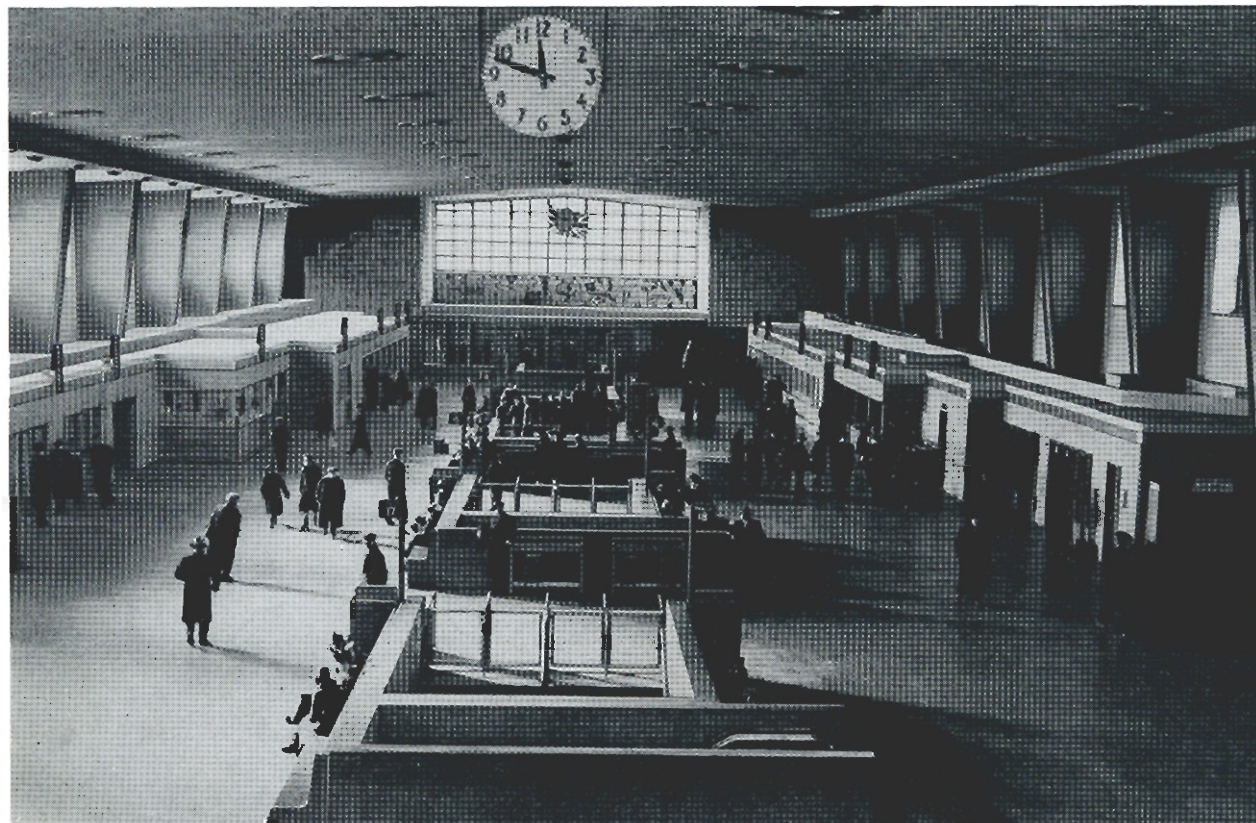
This view shows approximately one-half of the concourse. The entrance to the restaurant is seen in the background of the photograph; down the centre are the stairways and escalators joining the concourse and the train platforms.
