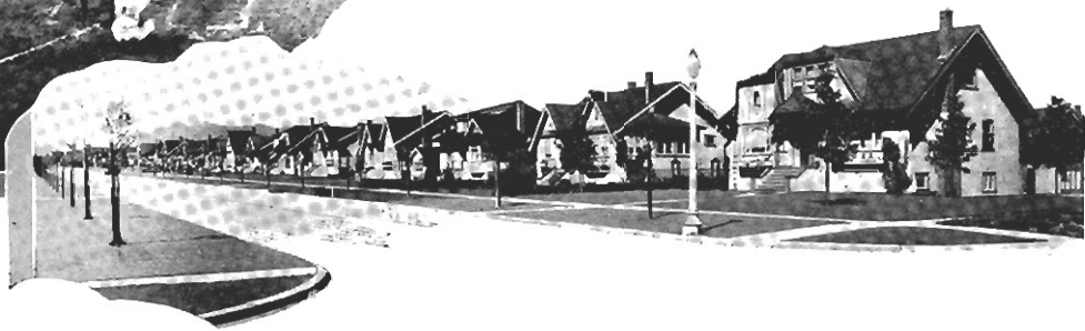
Top: Neon and flood lighting of the company's Granville street store building, Vancouver. Centre: Night baseball, Vancouver, made possible by flood lighting of park by company's engineers. Bottom: "From bush to residential street in two years"—two solid blocks of all-electrical homes, Vancouver.
