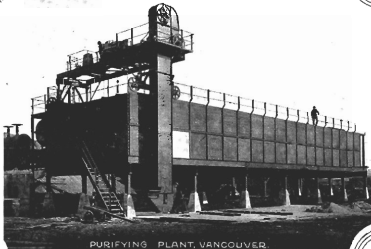
PURIFYING PLANT, VANCOUVER.
