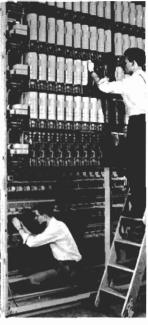
Since 1945 we have added about 2¼ million miles of wire and installed enough dial equipment to serve 423,000 telephones. Today, three-quarters of our customers have dial service. Careful planning, research, engineering and technical skill go into building and installing complex telephone equipment.
