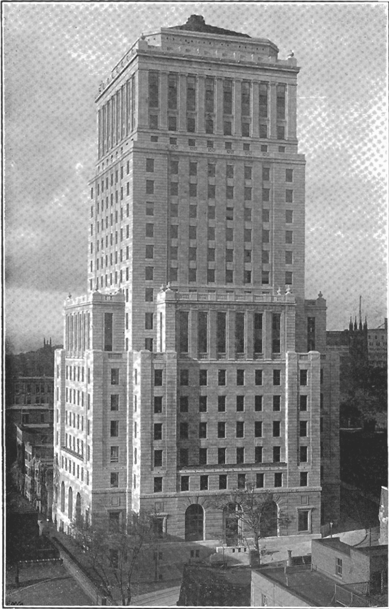
BEAVER HALL HEADQUARTERS BUILDING, MONTREAL
