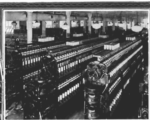
HIGH SPEED TWISTERS MAKING HIGH TWIST YARNS FOR BELDINGS AND CORTICELLI SILK HOSIERY
