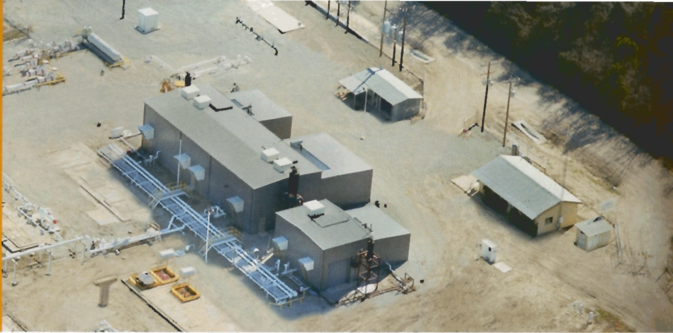
ATCO Noise Management constructed two acoustic buildings over three existing reciprocating engines and compressors at the Morgan Mill, Texas natural gas compression station, reducing noise levels to 47 dBA 750 feet from the centre of the plant.
