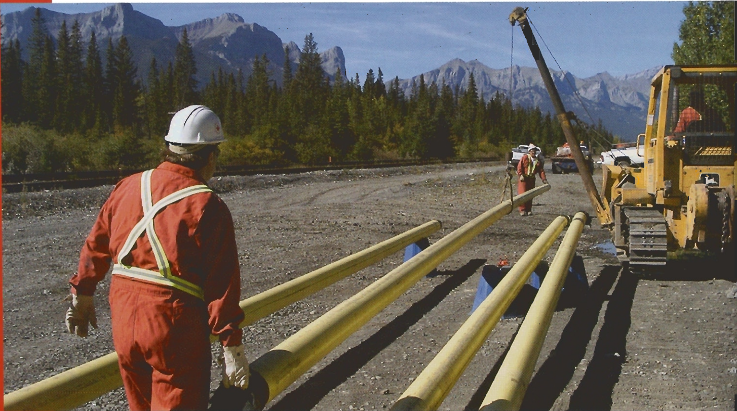
ATCO Pipeline installation near Exshaw, Alberta
