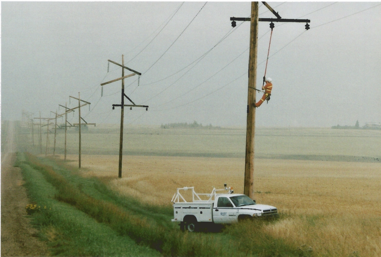
ATCO Electric Lineman
