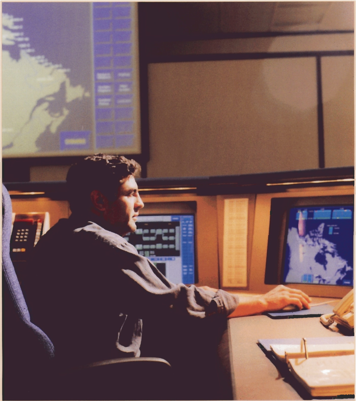
Remi Bisson, control centre technician, sits at the panel for supervisory control and data acquisition (SCADA) to remotely diagnose the radars in the North Warning System. The contract to operate and maintain the 47 radars and 5 logistics support sites of the North Warning System, held jointly with Pan Arctic Inuit Logistics Corporation, has been extended for 18 months to September 30, 2001.
