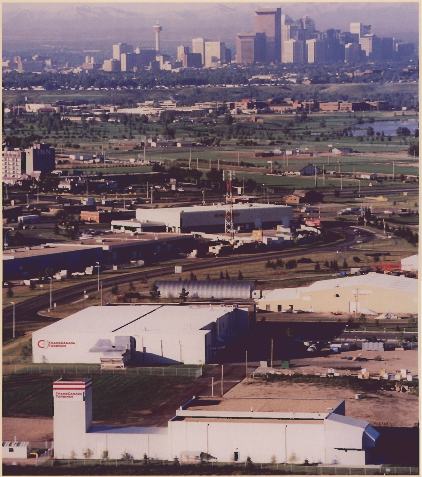
A significant highlight was the successful installation of the acoustic components, including inlet plenum and intake silencer, test cell liner, equipment door, augments tube, diffuser basket, and exhaust stack with silencer, for TransCanada Turbines Ltd.'s testing facility at Calgary, Alberta. The acoustic treatment of the turbine test cell represented a new market for ANM—one that is expected to grow along with turbine sales and maintenance requirements.
