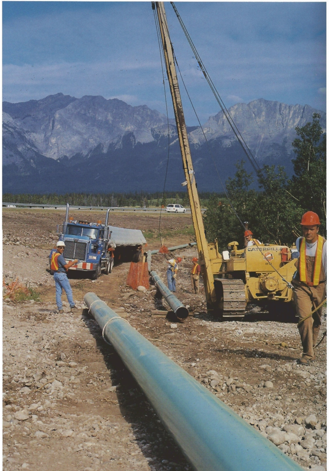
Banff Pipeline Looping Project, Summer 1998.
